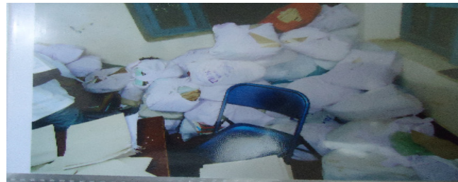
Figure 1. Poor Maintenance of Record Room.
