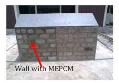
Figure 8. Micro-Encapsulation Wall.
