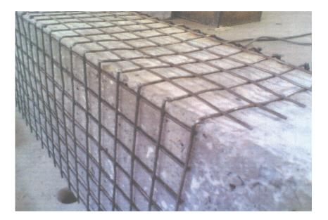
**Figure 4.** Application of welded mesh wire.
