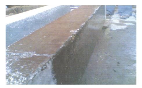
**Figure 3.** Application of bonded agent (epoxy).
