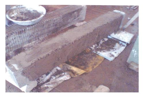
**Figure 5.** Application of cement mortar (15 mm thick).
