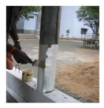
Figure 6. Columns over lapping with GFRP.
